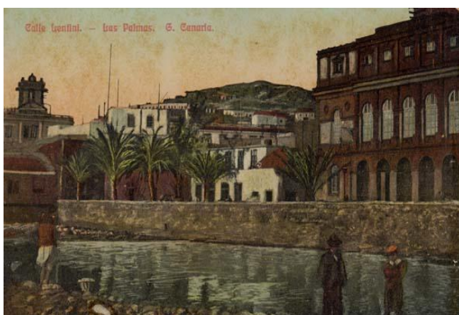
Calle Lentini along the barranco Guinguada, 1910. Source: FEDAC. Don Miguel's shop is located in the first building to the right.
