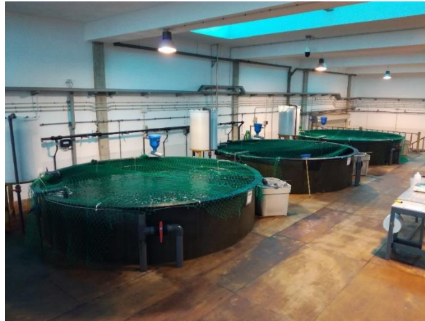
Figure 2-1. Tanks of 40 m 3 used along the studies of this thesis.
