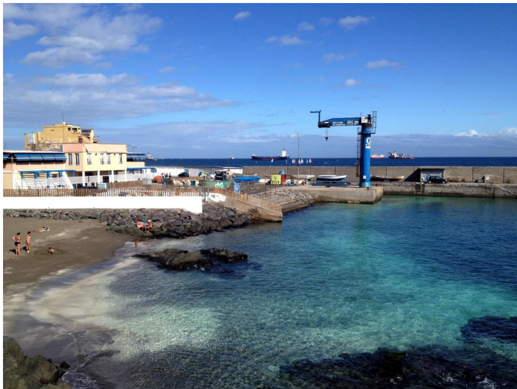
Photo 1. Current infrastructure of the fishing neighborhood of San Cristóbal (Author: Christian Linder Pons).
