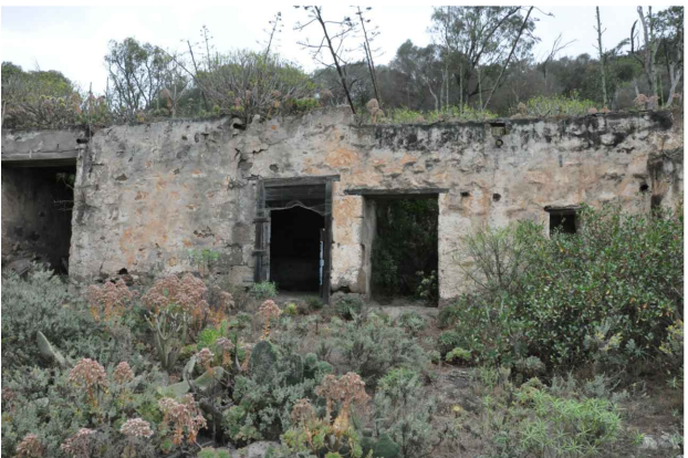
Vista exterior frontal del cuerpo E Frontal exterior view of the part E
