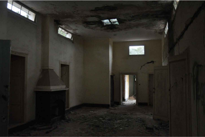
Vista interior del hall Interior view of the Hall
