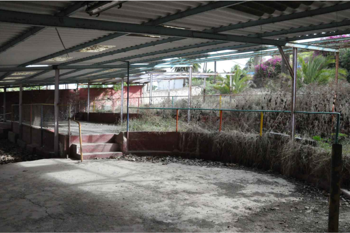
Vista interior espacio central Interior view central space
