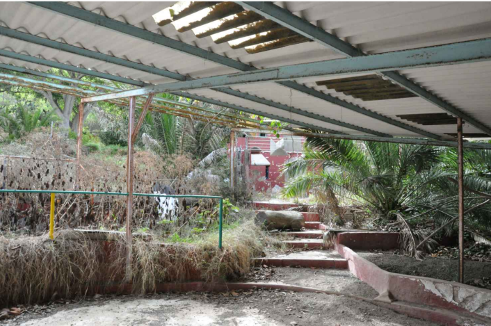
Vista interior espacio central hacia el patio interior Interior view central space towards the inner courtyard
