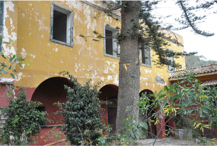
Vista general del cuerpo C General view of Part C
