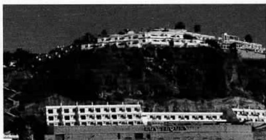
Figure 2. General view of Los Teques apartments and rocky slope in Southern Gran Canaria Island.
