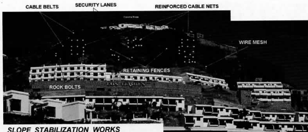
Figure 5. Stabilization methods used on Los Teques slope.
