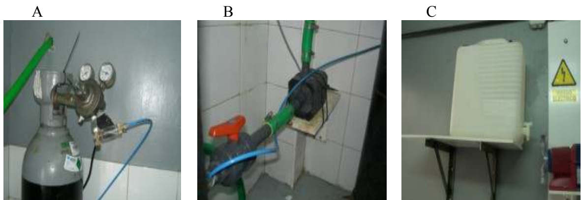
Figure 19. A. CO 2 gas cylinder with the electro-valve and plastic hose on the gas outlet. B. Plastic hose from the CO 2 electro-valve connected to the water pipe after the black tank and before the water pump. C. Enriched water plastic container connected to the peristaltic pump which leads the water to the fiber glass tank.
