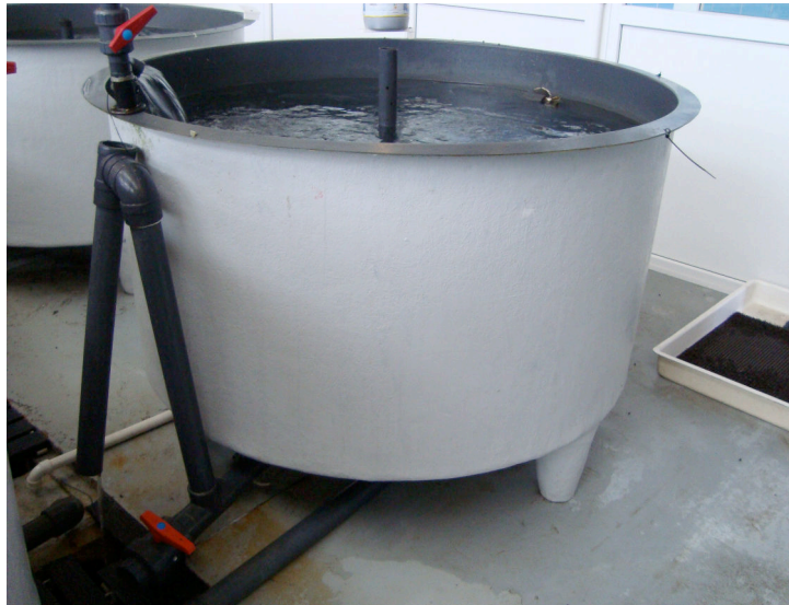
Figure 2.1: A 1000 l acclimatization tank
