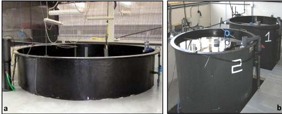
**Figure 18 (a, b).** a) Semi-intensive 40m<sup>3</sup> tank; b) Intensive 2m<sup>3</sup> tank.
