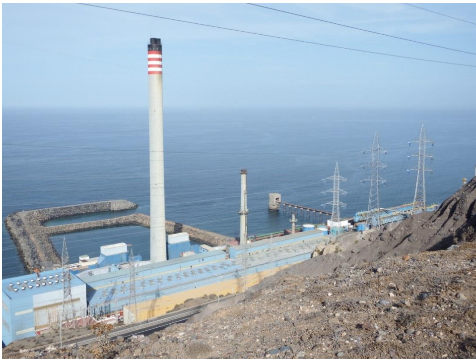
Thermal power plant. Jinámar, Gran Canaria, Canary Islands.
