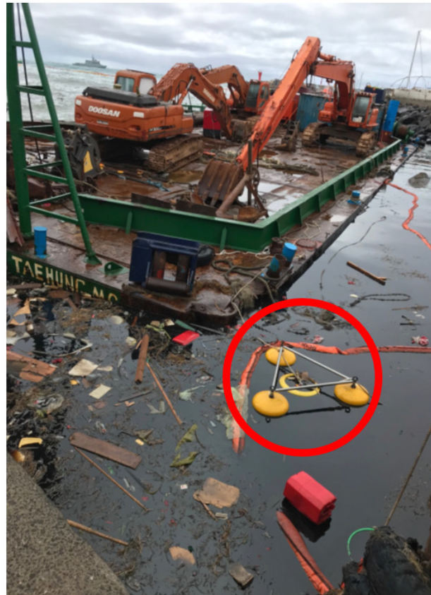
Figure 4. Standard Skimmer working (red circle).
