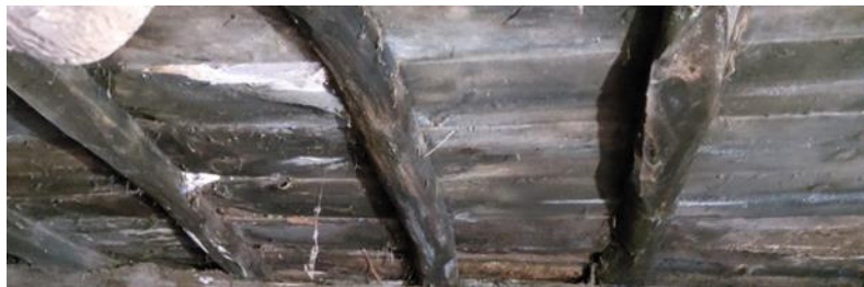
Figure – Example of a traditional timber pavement of Pedras Salgas Village
