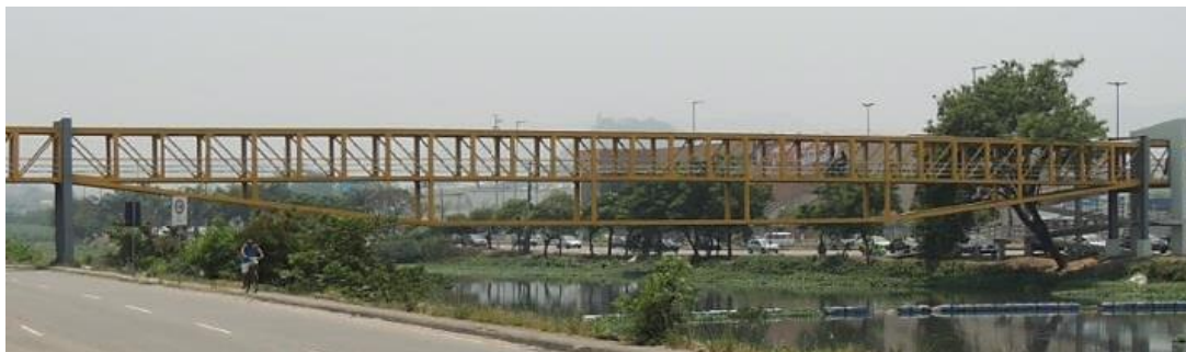
Figure 3: Inverted-queen-post-truss steel footbridge: FB-II ( L = 68.6 m).
