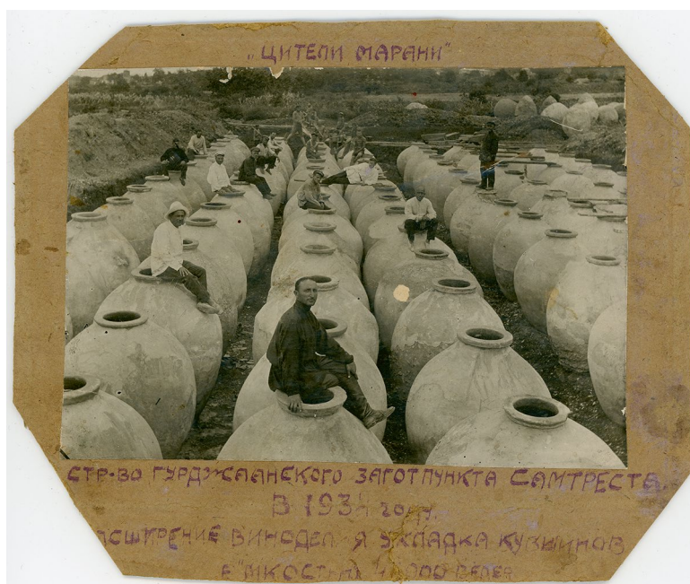
Fig. 14.3 Gurjaani, Kakheti. 1934. Inscription in Russian at the edge of the photograph: “‘Tsiteli marani’ [Red Cellar]. Construction of the ‘Samtrest’ supply station in Gurjaani in 1934. Enlargement of the cellar and installation of kvevris with a capacity of 4,000 buckets.” This cellar, with a total of 240 kvevris, is now owned by the large wine company Bolero & Co. (Source: © Luarsab Togonidze Private Collection)
