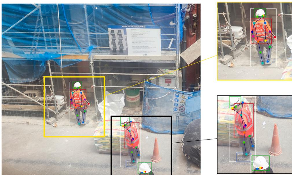
Fig. 4. Results for worker and PPE detection and matching in challenging scenarios: medium distance and minimally visible worker. Whole scene (left) and enlarged areas (right).
