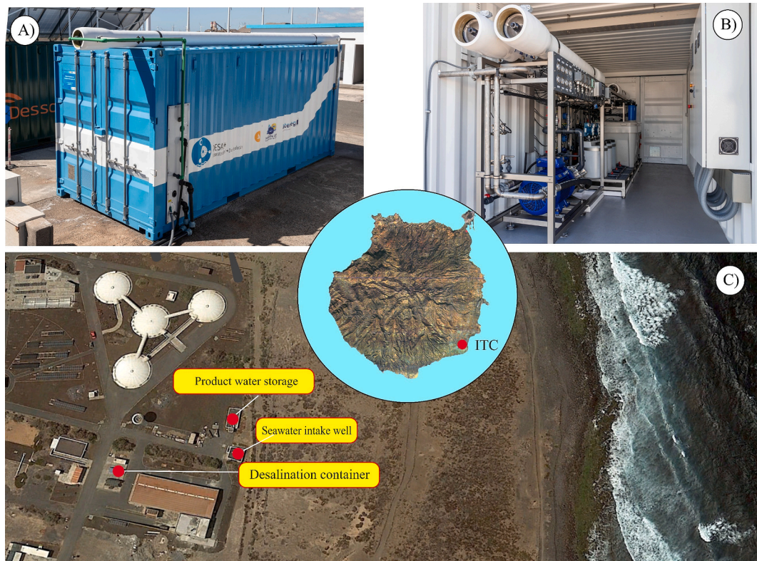
Fig. 2. A) Container housing the plant, B) Inside view of the container, C) Location of product water storage tank, seawater intake well and desalination plant container at the ITC premises.
