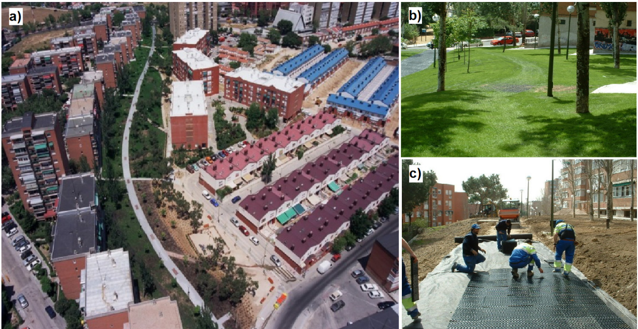
Figure 15. Gomeznarro Park [71]. (a) General view; (b) Finished pervious pavement; (c) Construction of pervious pavement.
