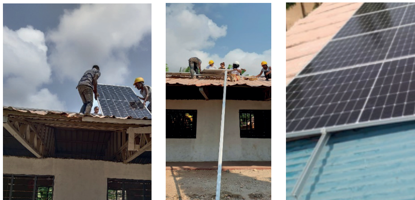
Figure 2. Installation of the solar panels on the roof of the building in progress.
