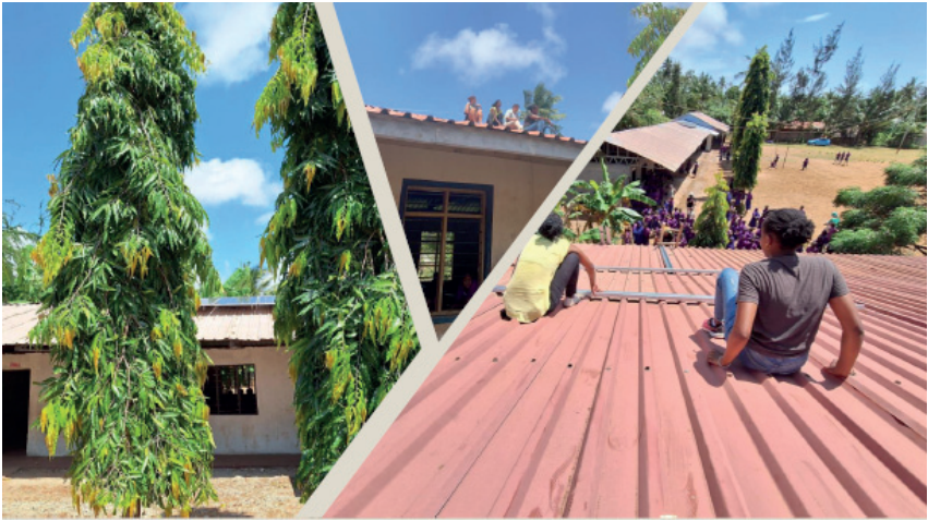
Figure 5. Installation of the solar panels for driving the water pump.
