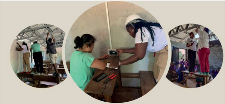
Figure 3. Installation of the lighting infrastructure.
