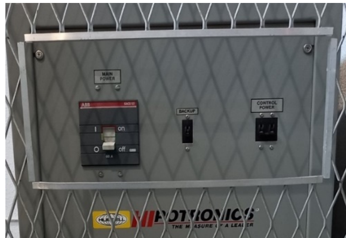
Figure 2. Power supply for the regulation of the output voltage, from 0 to 230 V.
