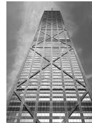
EDIFICIO JOHN HANCOCK CENTER, (CHICAGO 1965/1969) CONSTRUIDO CON SISTEMA "TUBE IN TUBE"
