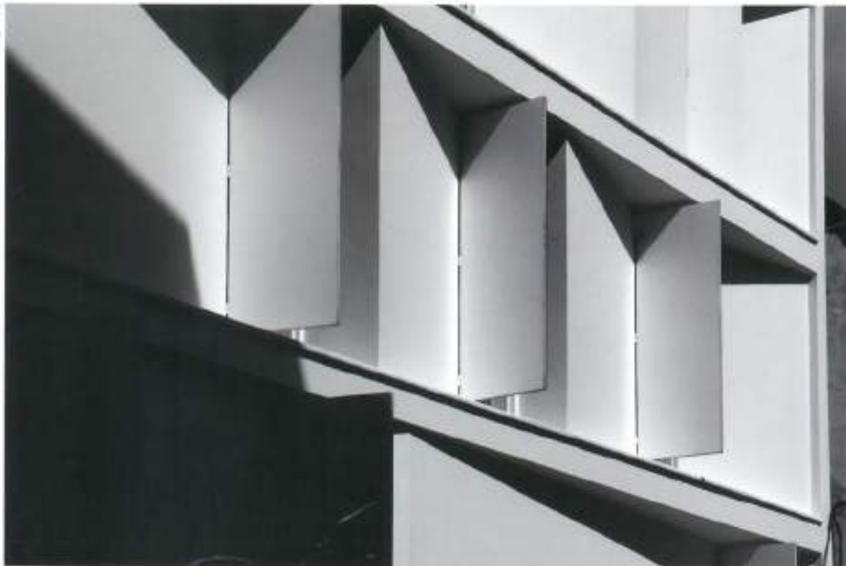
Open facade [detail view]
