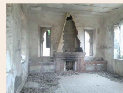
F5:Vista interior edificio dormitorios Interior views of dormitory buildings
