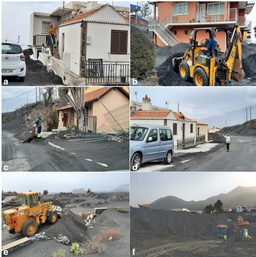
Fig. 15. Cleaning the thick lapilli deposits and reconstruction are the primary tasks after the eruption. a–d. Houses need to be cleaned and safety checked for structural damage and gas pockets and traps before populations can return to the properties that were not swallowed up by lava or collapsed under the weight of the ash. e, f. Transport of lapilli to temporary pile-up sites allow storage of large amounts of ash before being hopefully redeployed as concrete supplements, aggregates in road construction, and soil supplements in agriculture. Images are from San Nicolás and the Las Manchas region.
