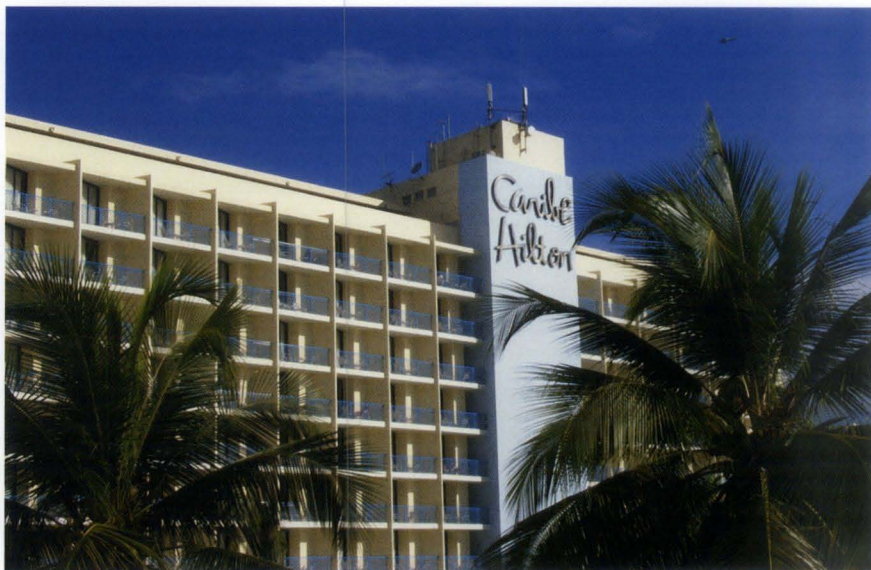
Fig. 2. The Caribe Hilton in San Juan (1945), designed by the San Juan architectural firm of Toro, Ferrer y Torregrosa. (Copyright free web image).
