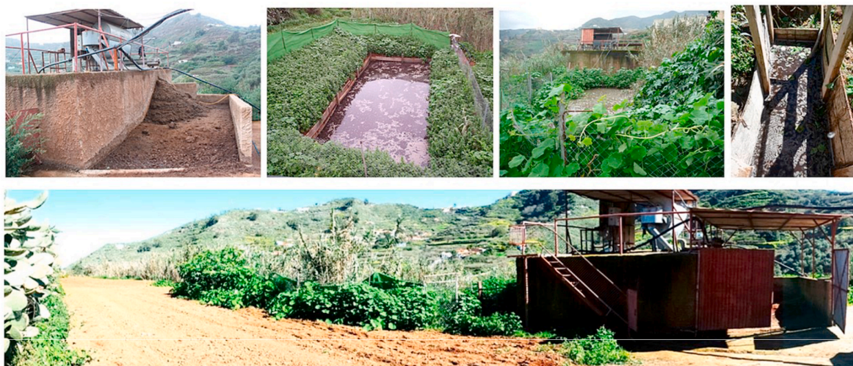
Fig. 2. From left to right: digester and rotary screen and solid, pond, constructed wetlands, final tank and (below) panoramic view.
