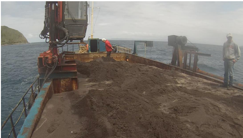
Figure 8. Visual Inspection on board when the sand filling is complete @ImagDOP.
