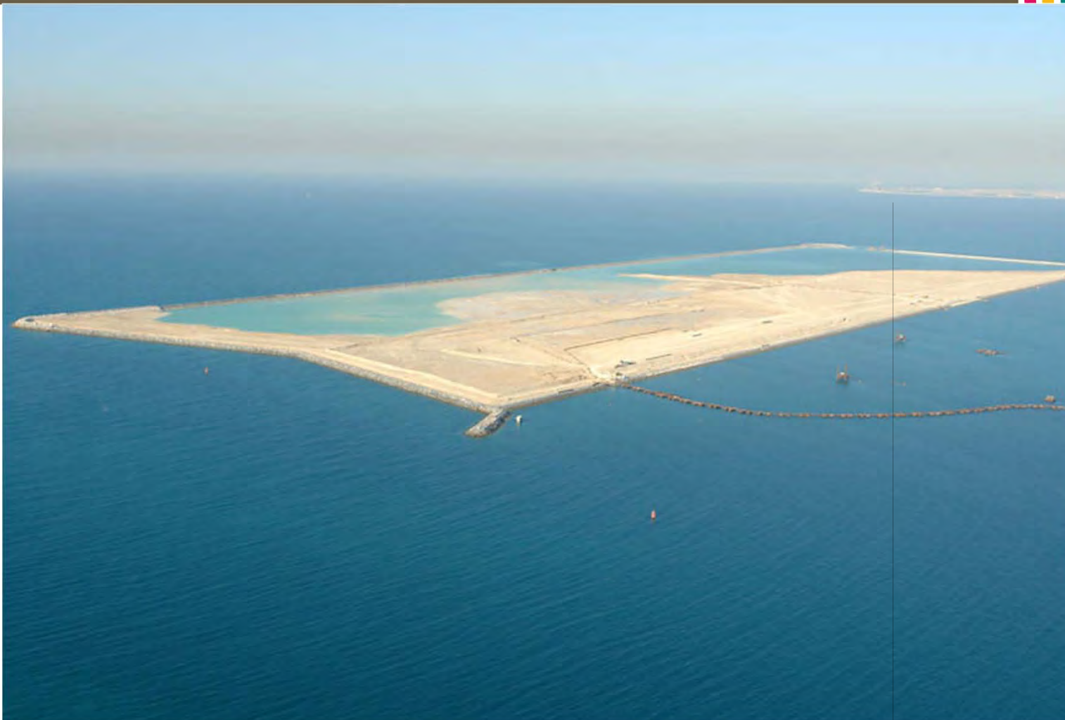
Jebel Ali New Container Terminal Stage 1 - Dubai (U.A.E.) | 2005-2009
