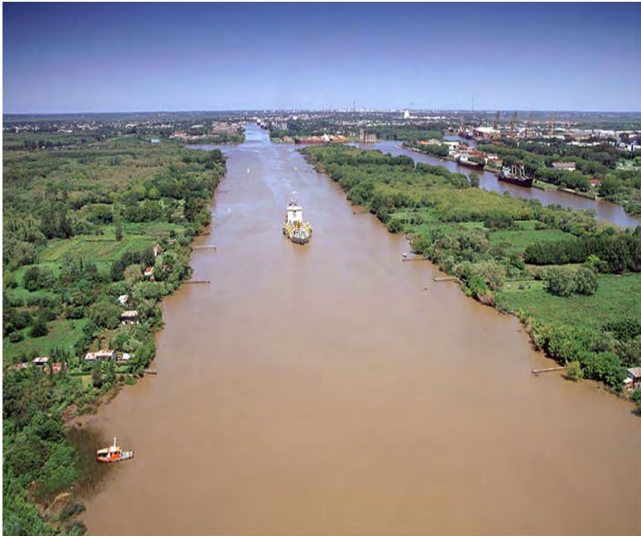
TSHD Captan Nuñez maintenance dredging
