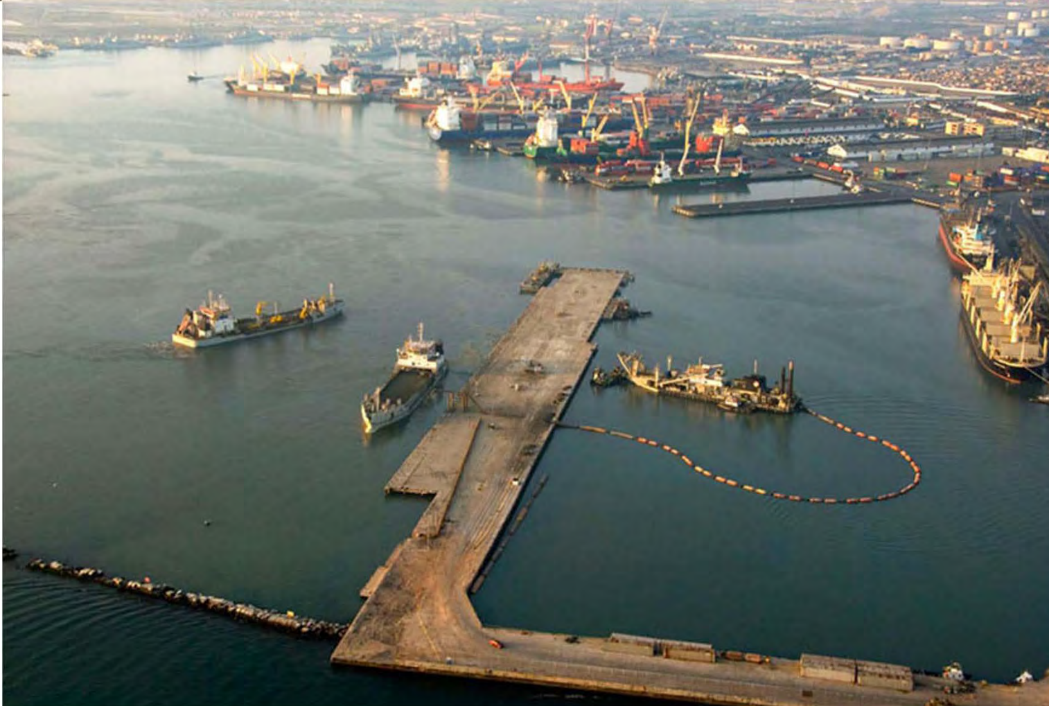
Callao Terminal - Peru | 2008-2010 Dredging: approx. 4,000,000 m 3 , Reclamation: approx. 2,000,000 m 3
