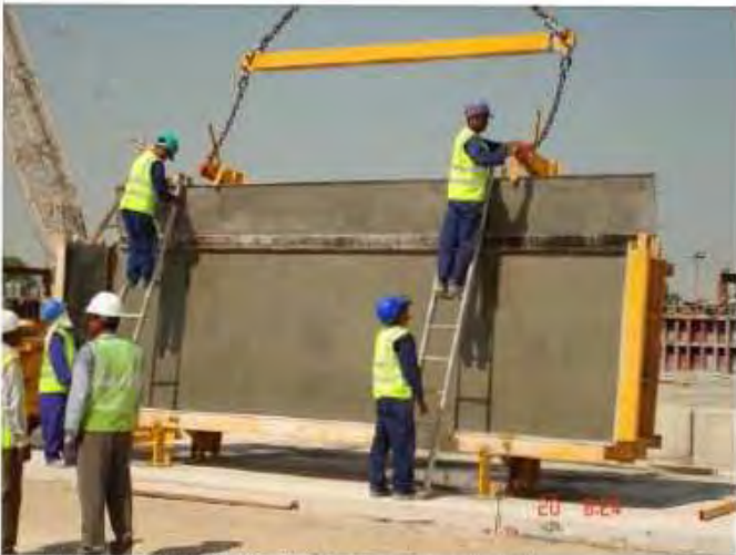
Formwork Course-4B, Precast Front Panel. Open position after removing block.
