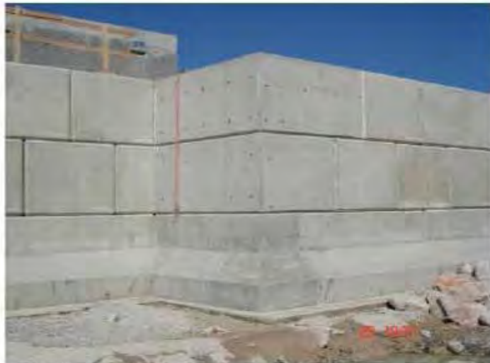
Insitu casted "Pontoon-Corner" after completion
