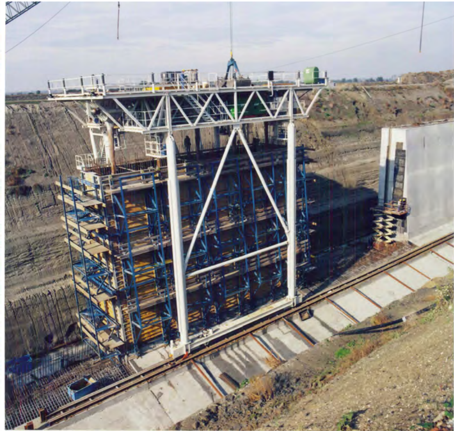
Sliding formwork
