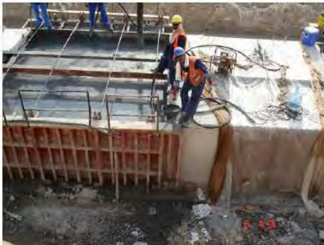
Course-1: casting 2-side mould
