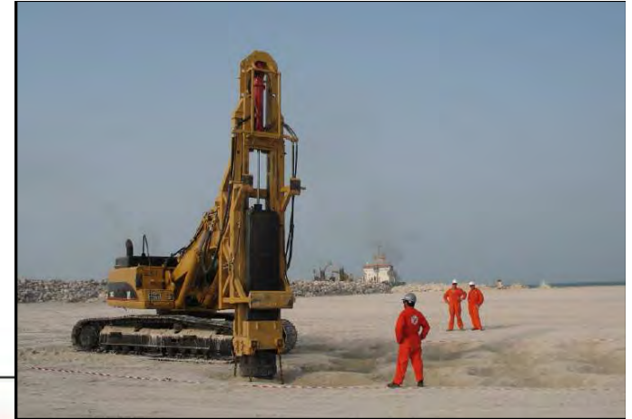
Rapid Impact Compaction (RIC), at Ras Laffan Port, Qatar
