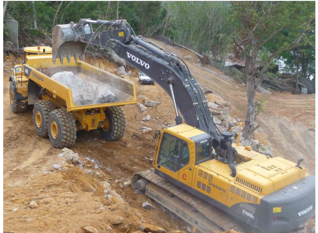
Loading & transport of blasted rocks
