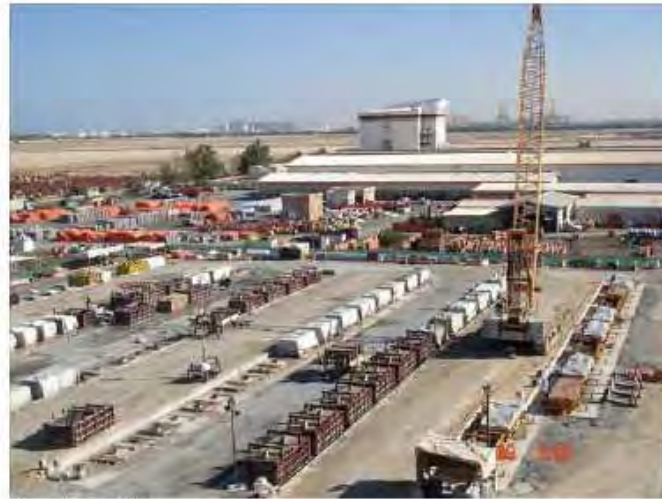
Overview Precast Yard
