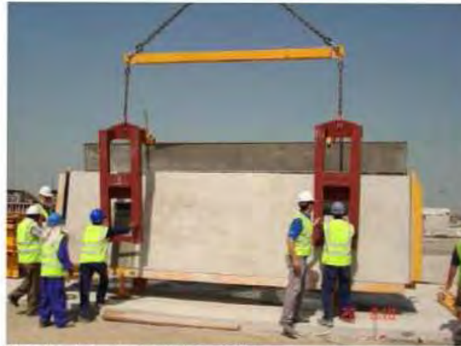
Course-4B "Precast Front Panel": Lifting block out of mould.
