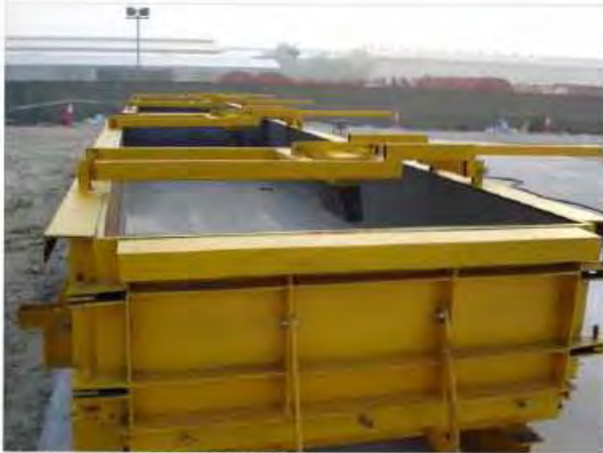
Formwork Course-4B, Precast Front Panel. Casting position.
