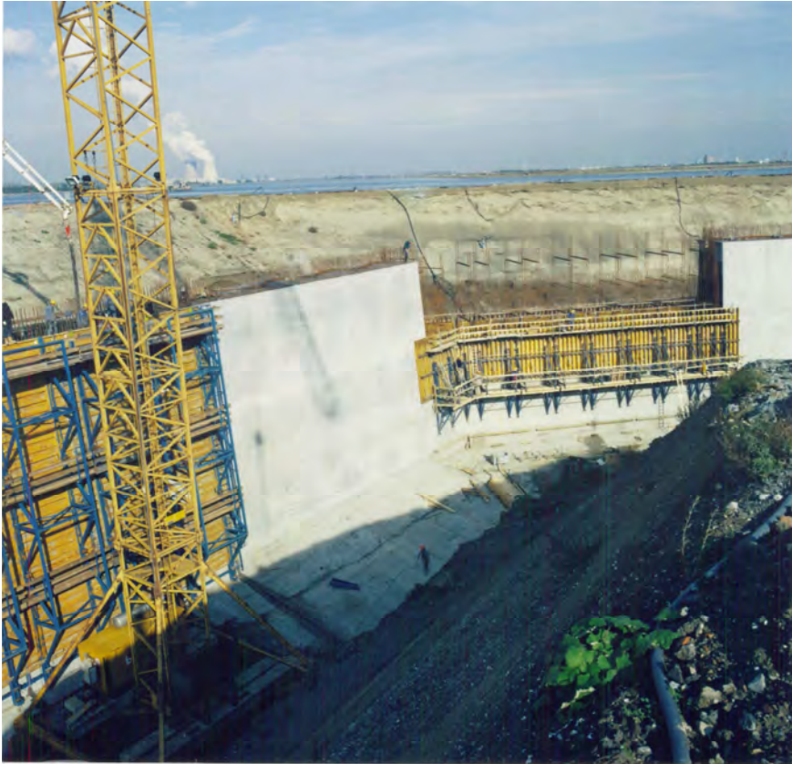
Fixed Formwork in corners
