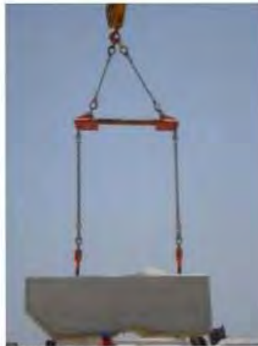
Lifting Course-2 block.
