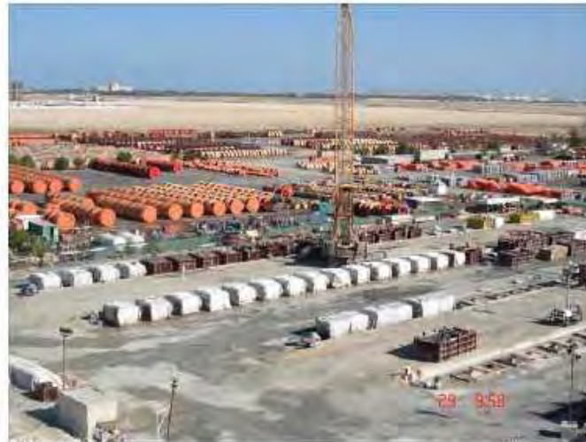
Overview Precast Yard
