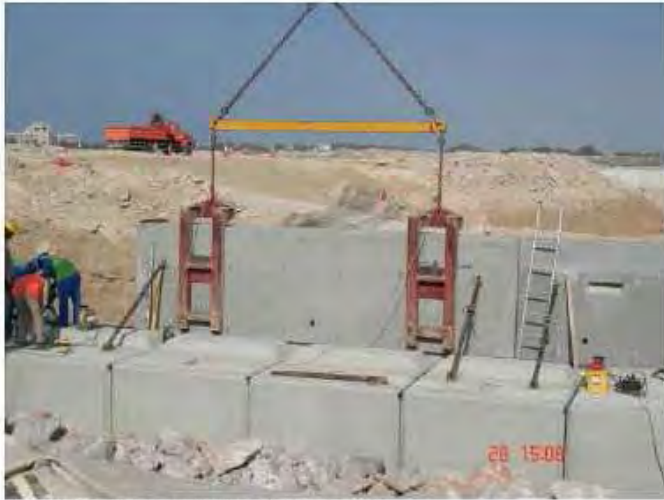
Course-4B "Precast Front Panel": Placing blocks at Quay Wall.
