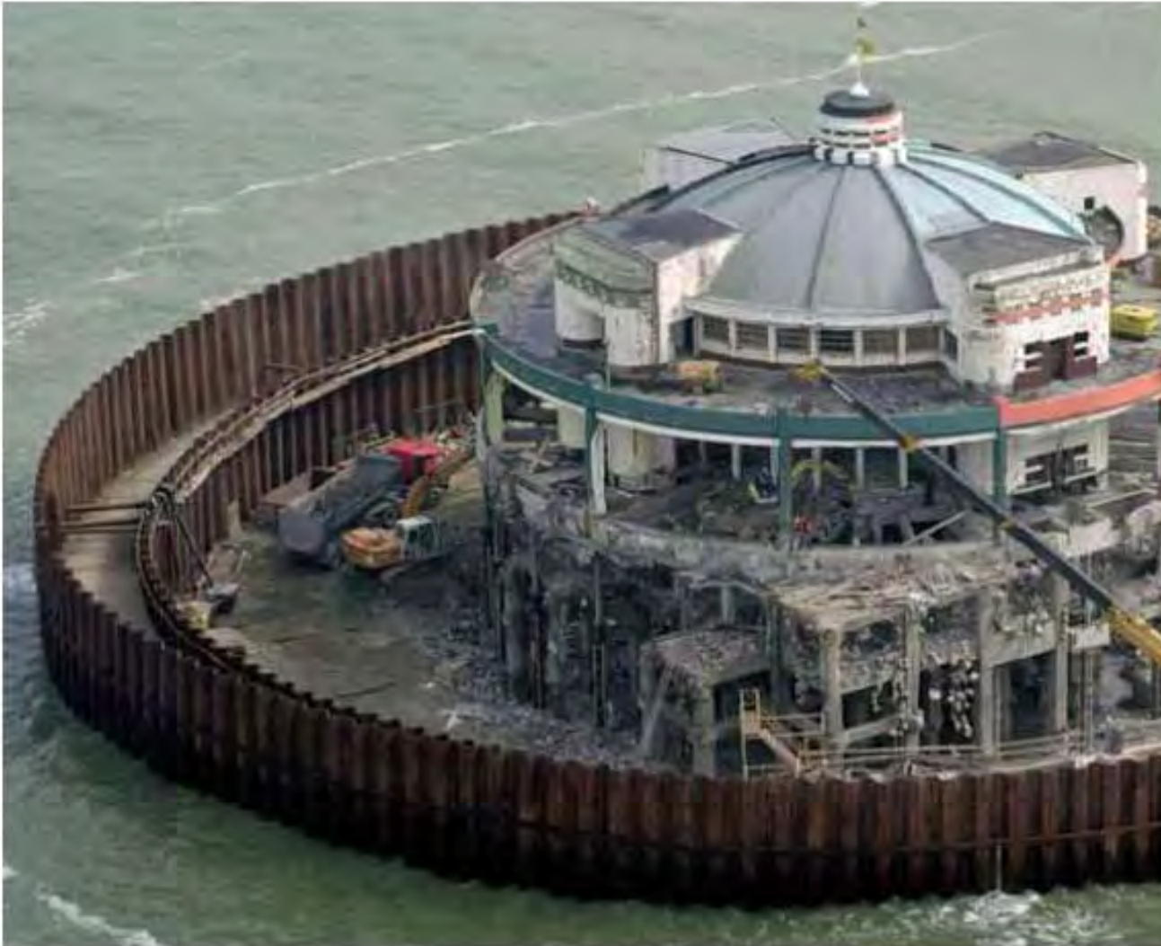
Double sheet-pile wall, Blankenberge (Belgium)
