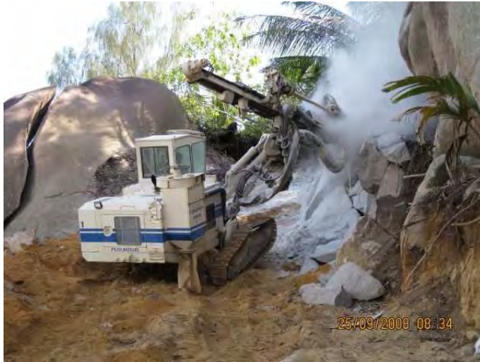
Jumbo-Drilling of drill-holes
