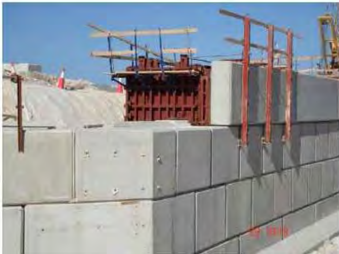
Course-4B "Precast Front Panel": Side view with mould Course-4A
