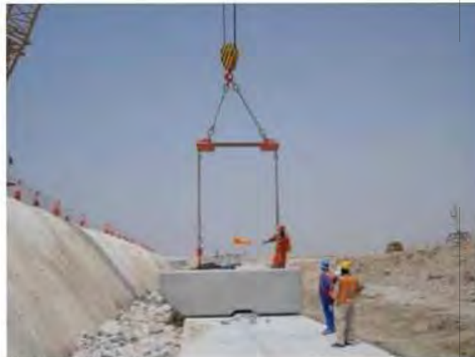
Placing course-2 block.
