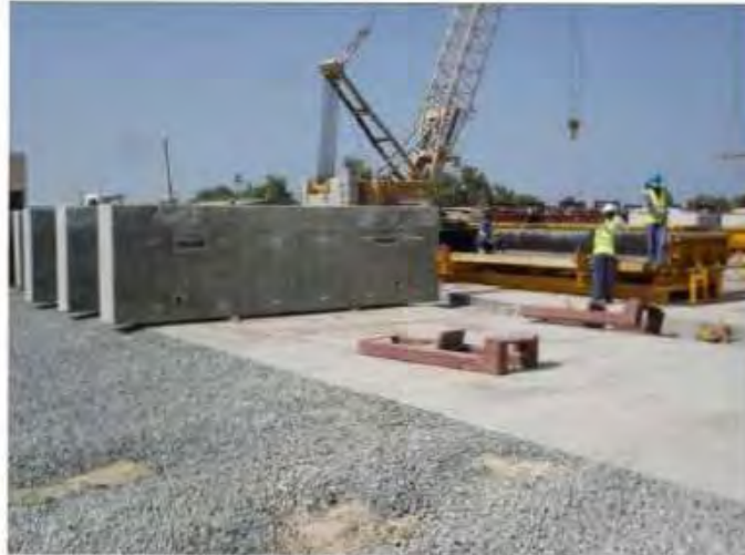
Course-4B "Precast Front Panel": Stockpile & GFRP-bars for connection with C4A.
