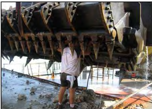
PHOTO 3: Vasco crew removing coral blocks between the ripper teeth.
